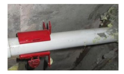
It goes without saying that the intumescent material must be left in the clamp, stripped out on these two clamps as the pipe joint makes it impossible to wrap the metal clamp around the pipe
