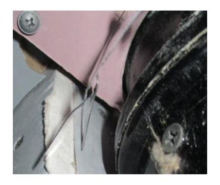
Wrapping two collars without securing them will just push the metal restraining rings away and not seal the pipe.
